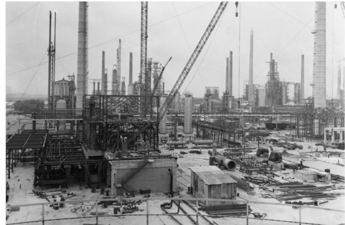
New oil refineries under construction at Pernis (Netherlands), 1967
