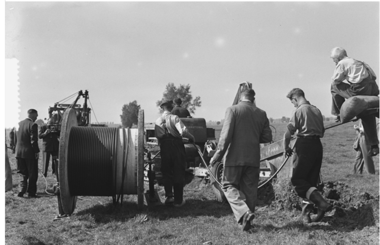
Laying plastic water supply pipes underground at Odijk, near Utrecht (Netherlands), 1953
