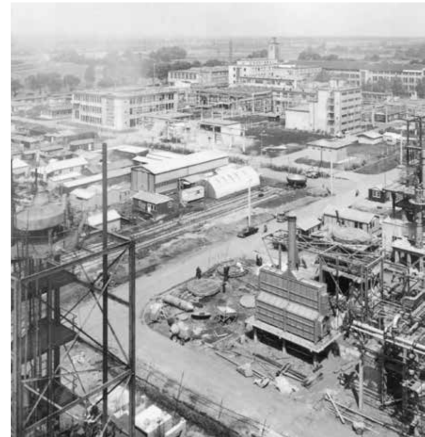
In 1963, DSM started construction work on a melamine plant. The buildings of the company's Central Laboratory are to be seen in the background.
