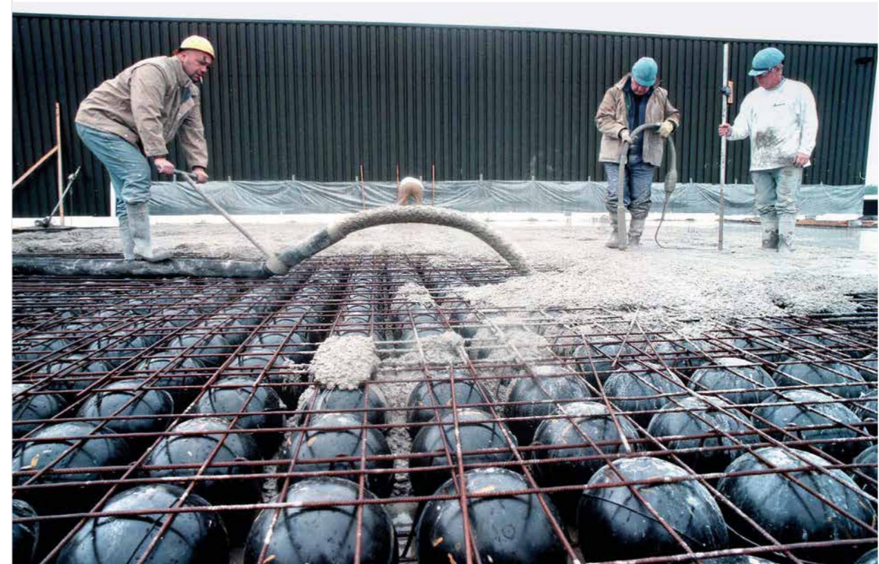
Builders working on a DubbleDeck floor in Arkel (Netherlands). DubbleDeck is a new, environmentally friendly concrete floor system developed by a Danish engineer. The system consists of a steel lattice incorporating large, hollow plastic balls, enabling a 35% materials saving on iron and concrete. The system was also used in the construction of the 35-storey Millennium Tower in Rotterdam.
