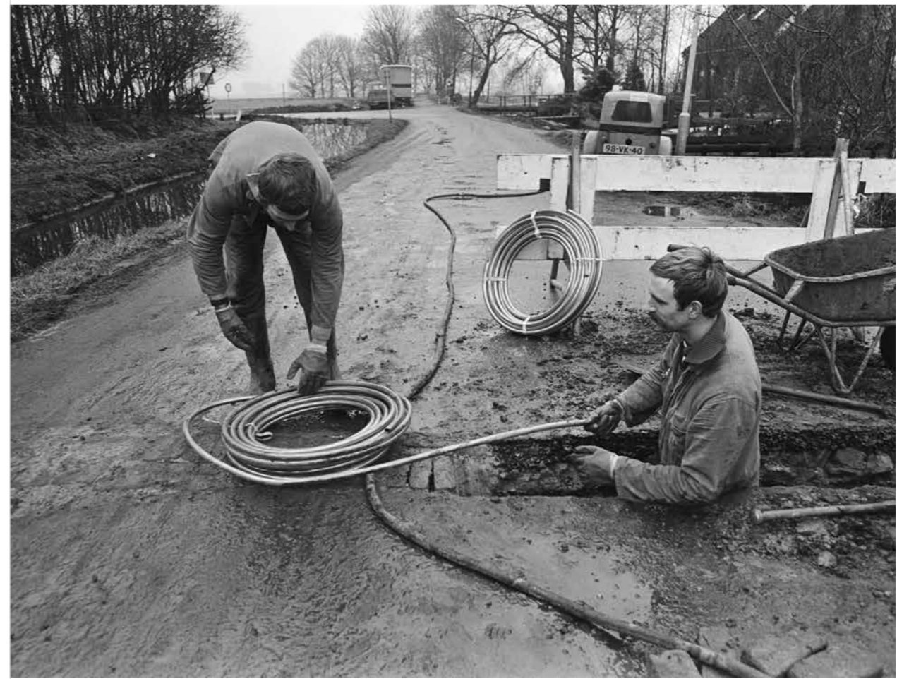
In the Dutch town of Broek in Waterland, PVC water pipes were replaced by copper pipes after toxic substances had been found in the drinking water (January 1981).
